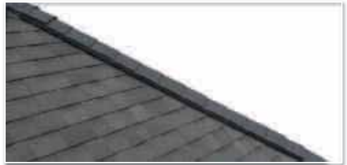
Hip Ridge Vent Installation
